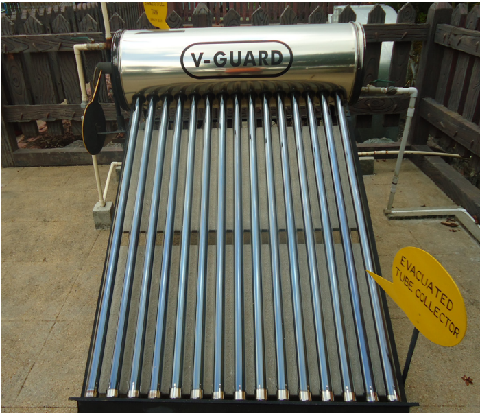
A solar water heater. Photo credit: RanjithSiji via Wikimedia Commons. CC BY-SA 3.0
