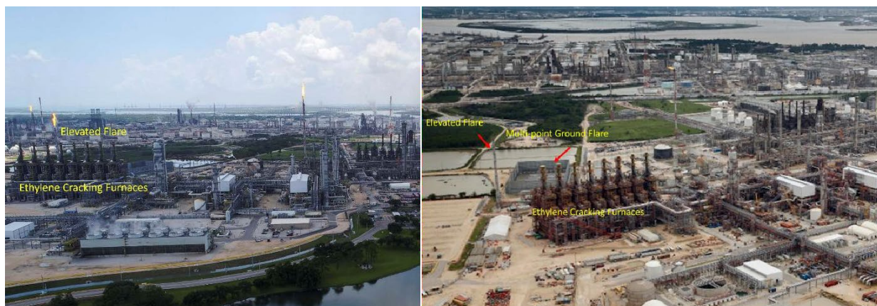
192 Figure 7 - Cracking furnaces with elevated flare and multi-point flare that treat waste gases from cracking system.
