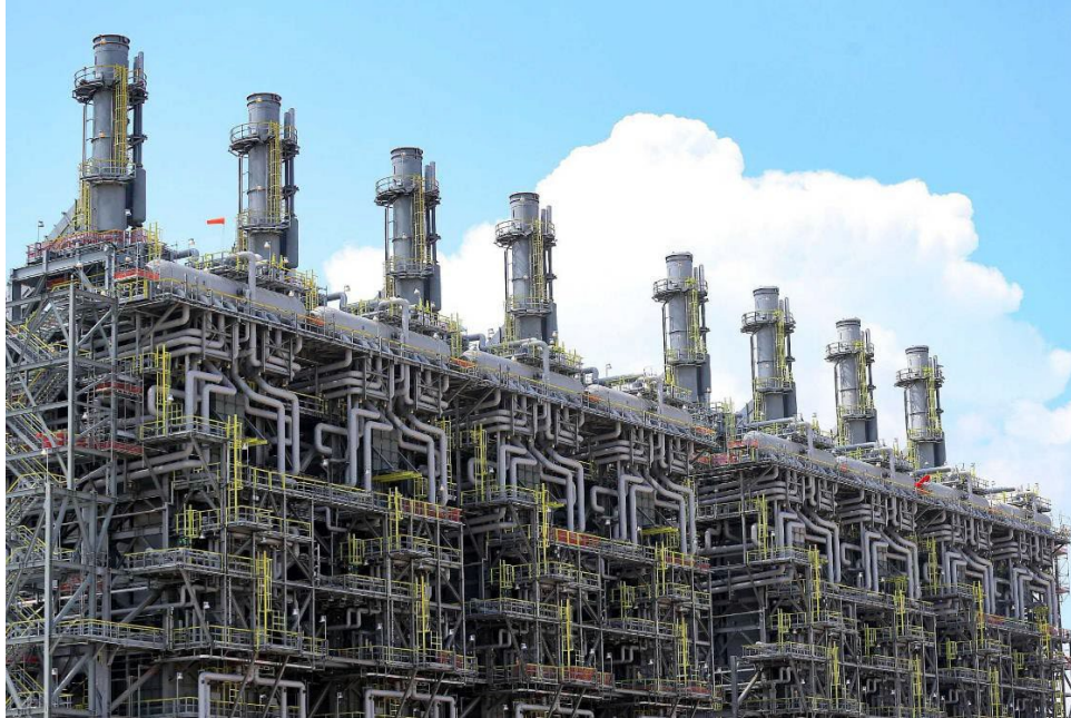
132 Figure 2 - Baytown ethylene cracker system at the EXXON Baytown refinery
