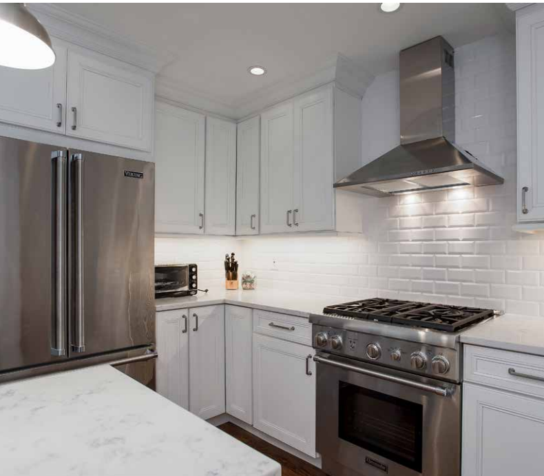
A gas stove with external ventilation.
